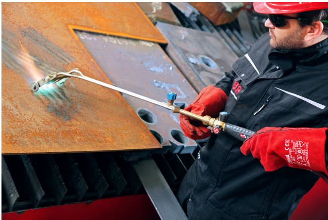
Straightening with GCE U7™ TORCH SYSTEM
