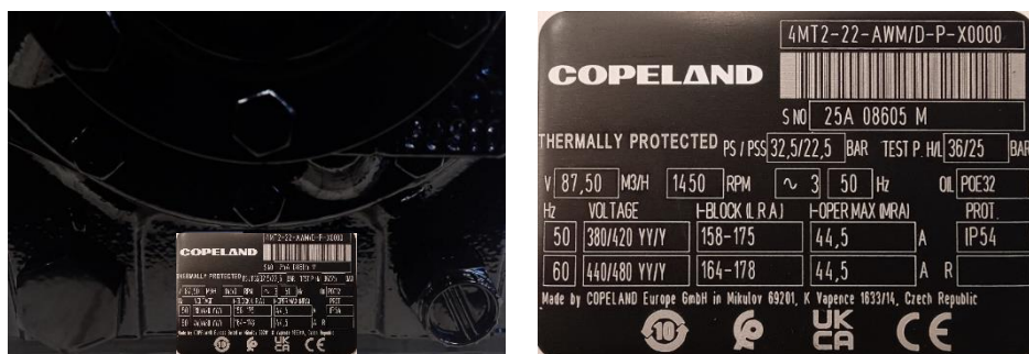
Figure 2: Stream compressor nameplate and nameplate location
